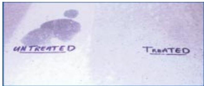
Test Areas Shown After Cleaning
